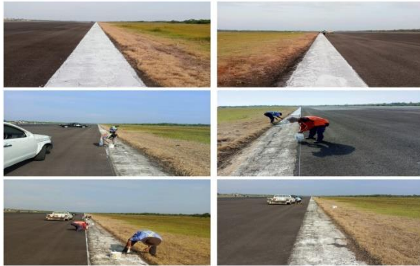
Gambar 4.4 Pengecatan Marka Runway Side
