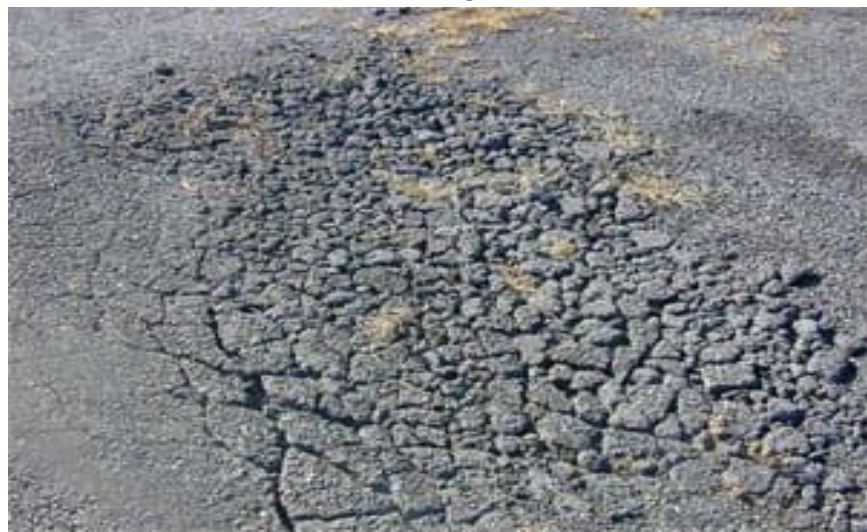
Gambar 2.1 Alligator Crack
