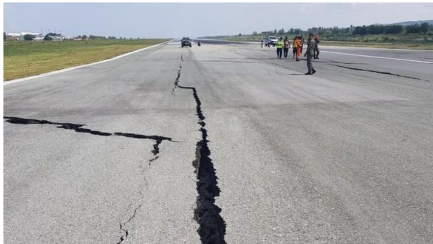
Gambar 2.2 Longitudinal Crack
