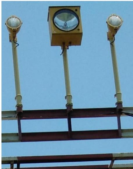
**Gambar 2.5 Sequence Flashing Light**
