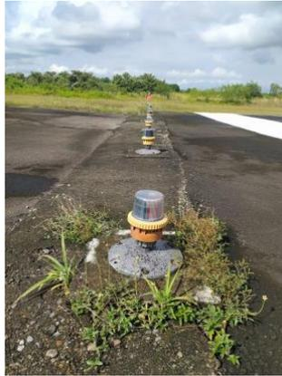
**Gambar 2.2 Lampu *Threshold/ Runway End Light***
