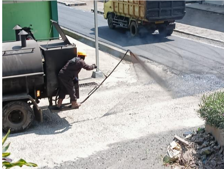
Gambar 4.16 Pekerjaan Prime coat
