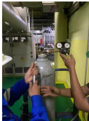
Gambar 4.5 Proses pengisian gas SF6
