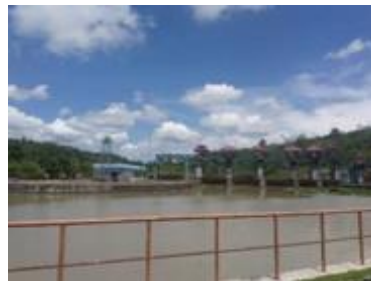
Gambar 2.2 intake dam PLTA Musi
